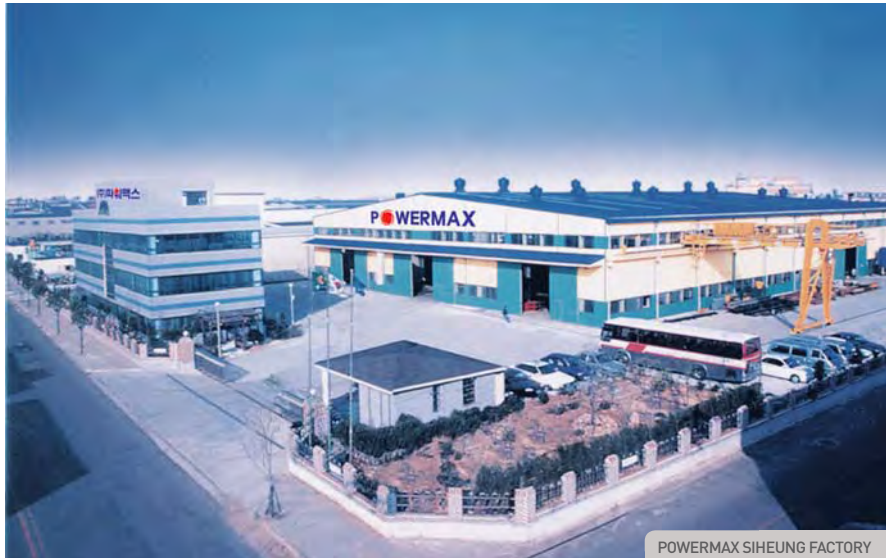
POWERMAX SIHEUNG FACTORY
